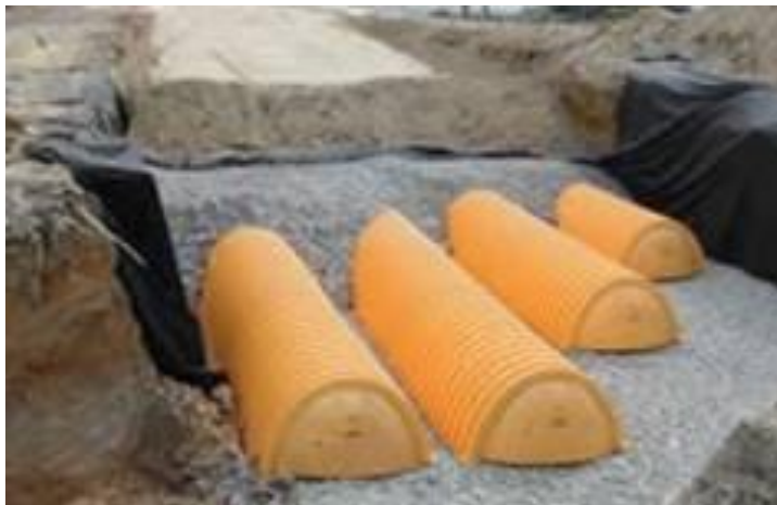
Devens Common underground infiltration systems
