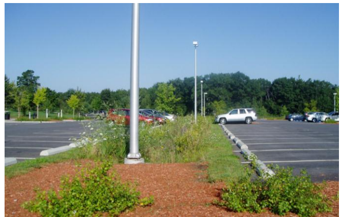
Low-Impact Development parking lot design (biofiltration)
